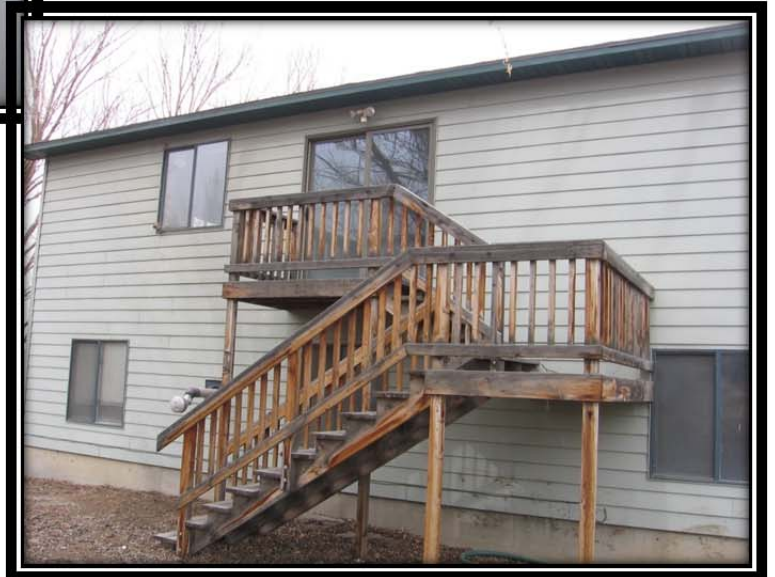
Stairs to Master Bedroom
